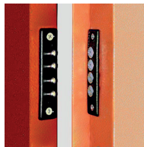
Electrical contacts between leaf and doorframe
